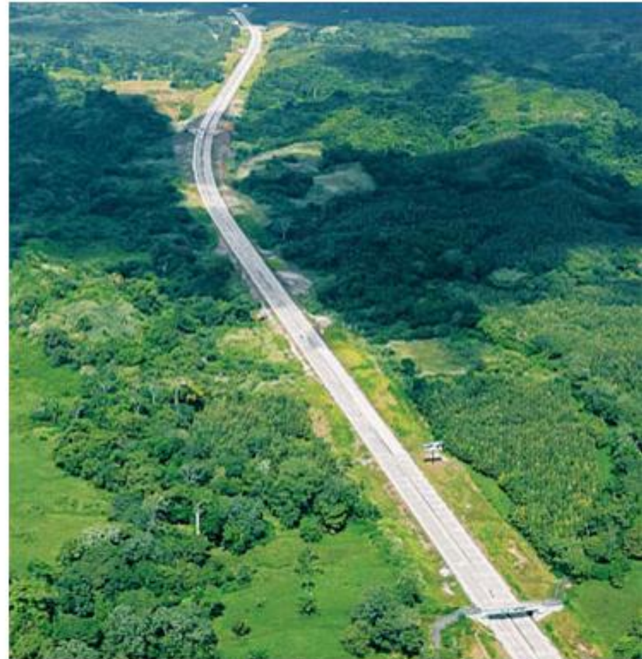
Alberto Motta Highway, Panama – CEMEX Conventional Concrete
